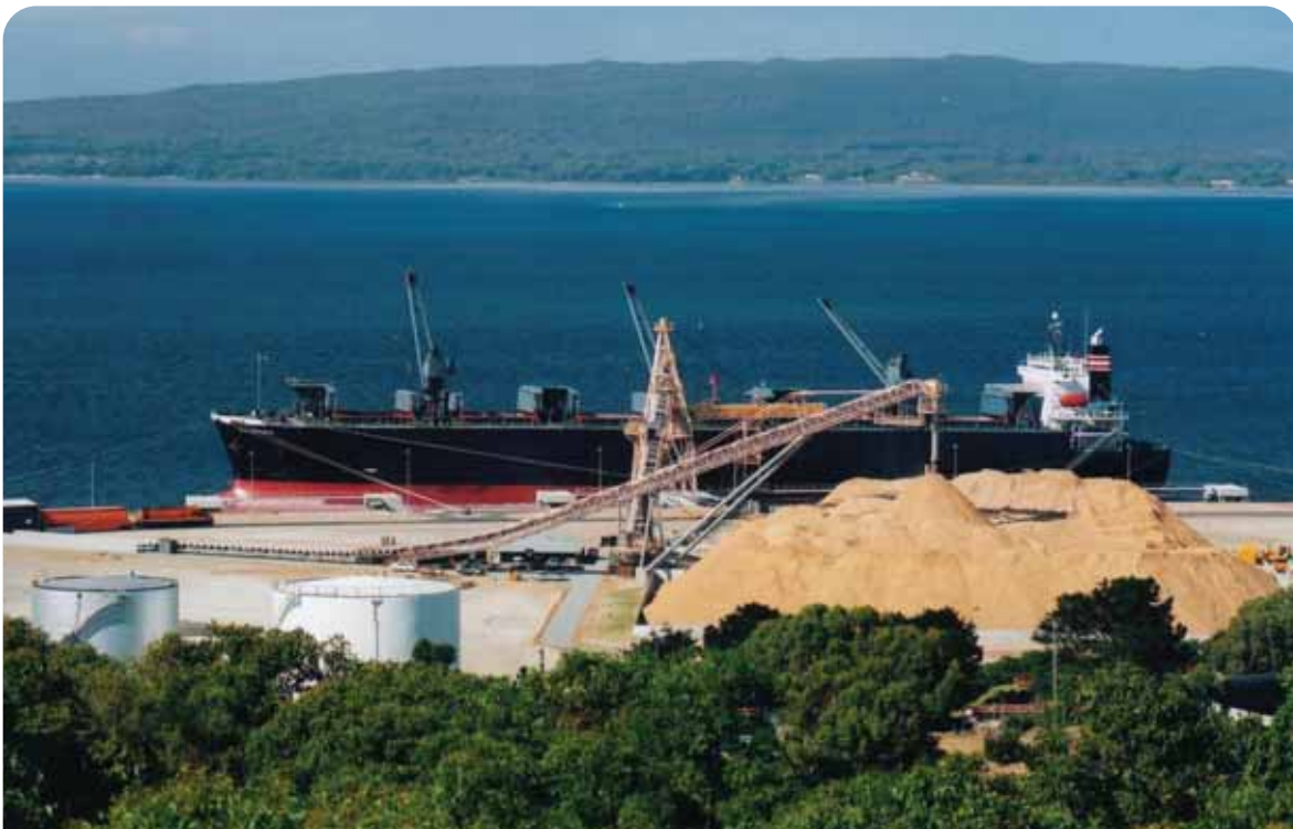
Albany and Bunbury have multiple hardwood chip and port facilities
